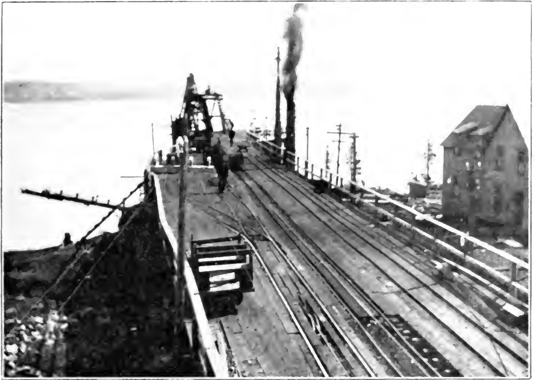
Trestle and Tipple over Storage Bin, at Wabana Iron Mines
